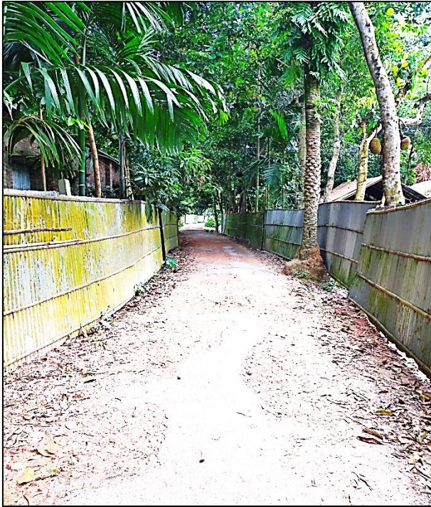
Road-1 + Drain-2, Ulipur Pourashava
